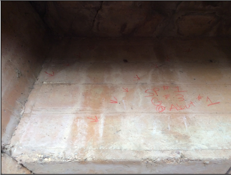
Span #1, girder #3 at abutment #1-Hairline shear crack.
