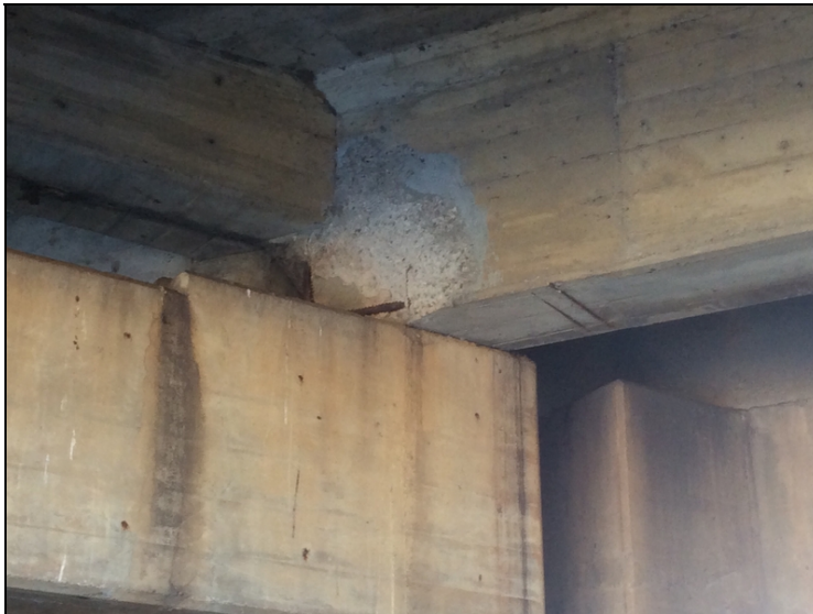
Span #1, Girder 3 over Bent 2-Spalling with exposed reinforcing steel.
