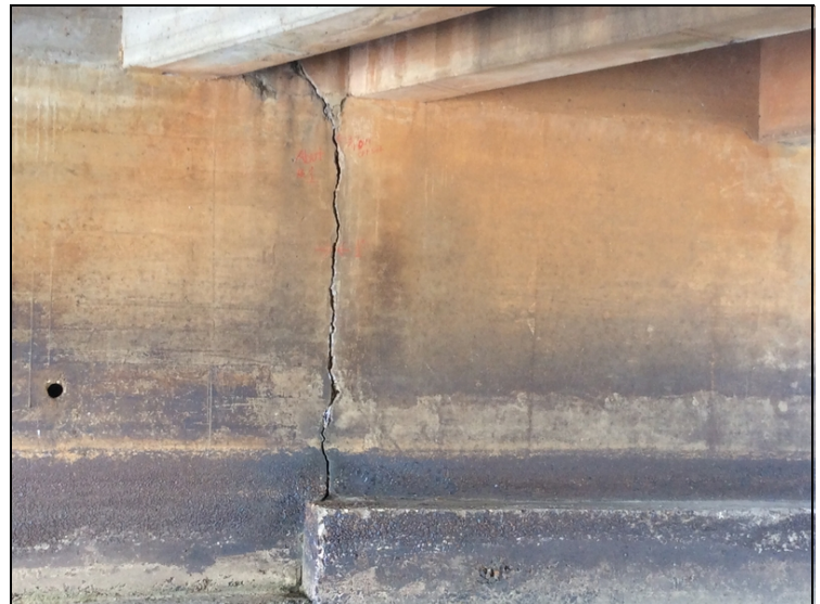
Abutment #1-Wide racking in breastwall at construction joint.
