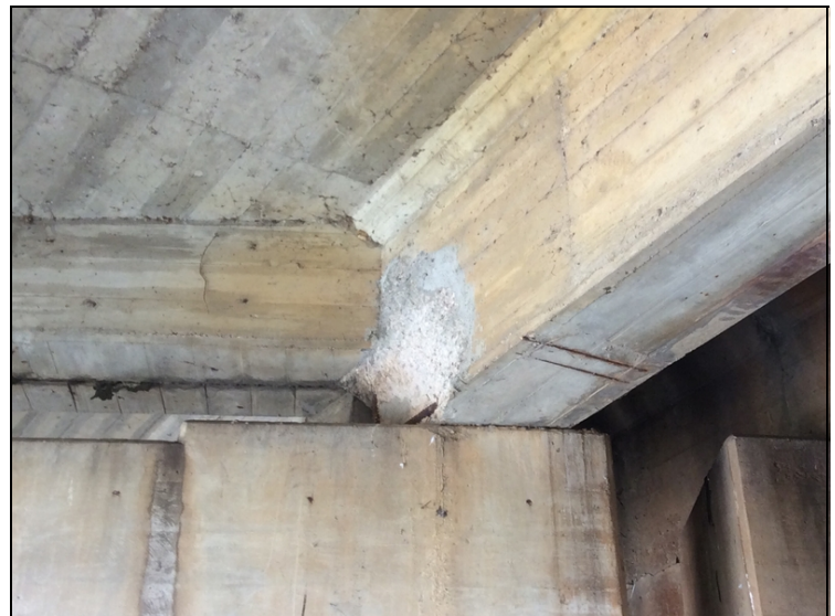
Spall with exposed reinforcing steel in Span 1. Girder 3. At Bent 2.
