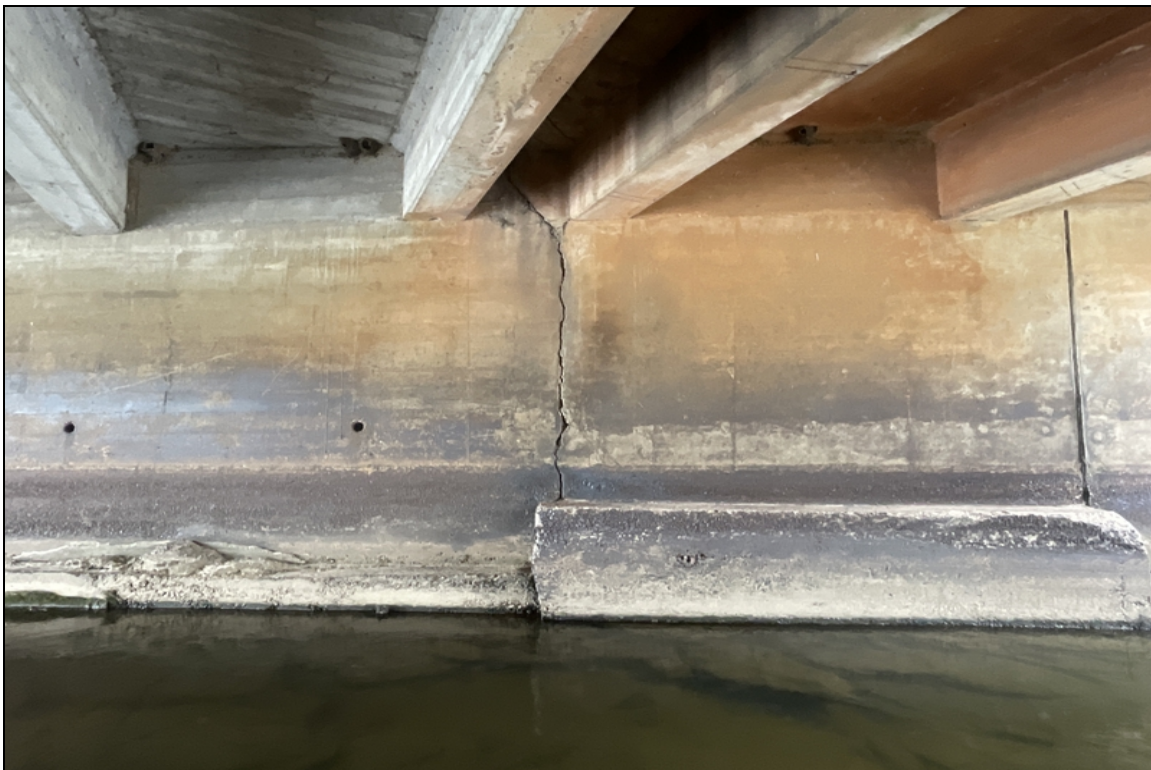
Bent # 1 stem wall appears to have rotated approximately 3/4" toward the channel at the construction joint in Bay # 3 under Girder # 3. The stem wall has a 1/2" wide crack at the construction joint with 3/4" differential offset at the crack.
