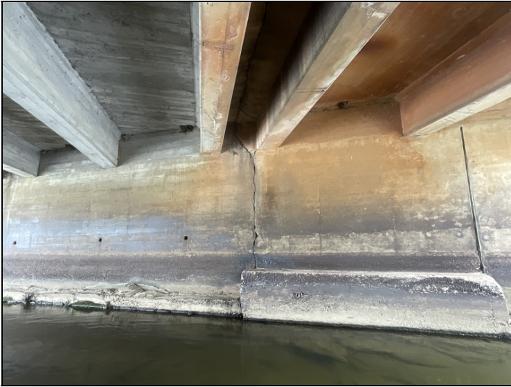
Bent # 1, Bay # 3 construction joint.
