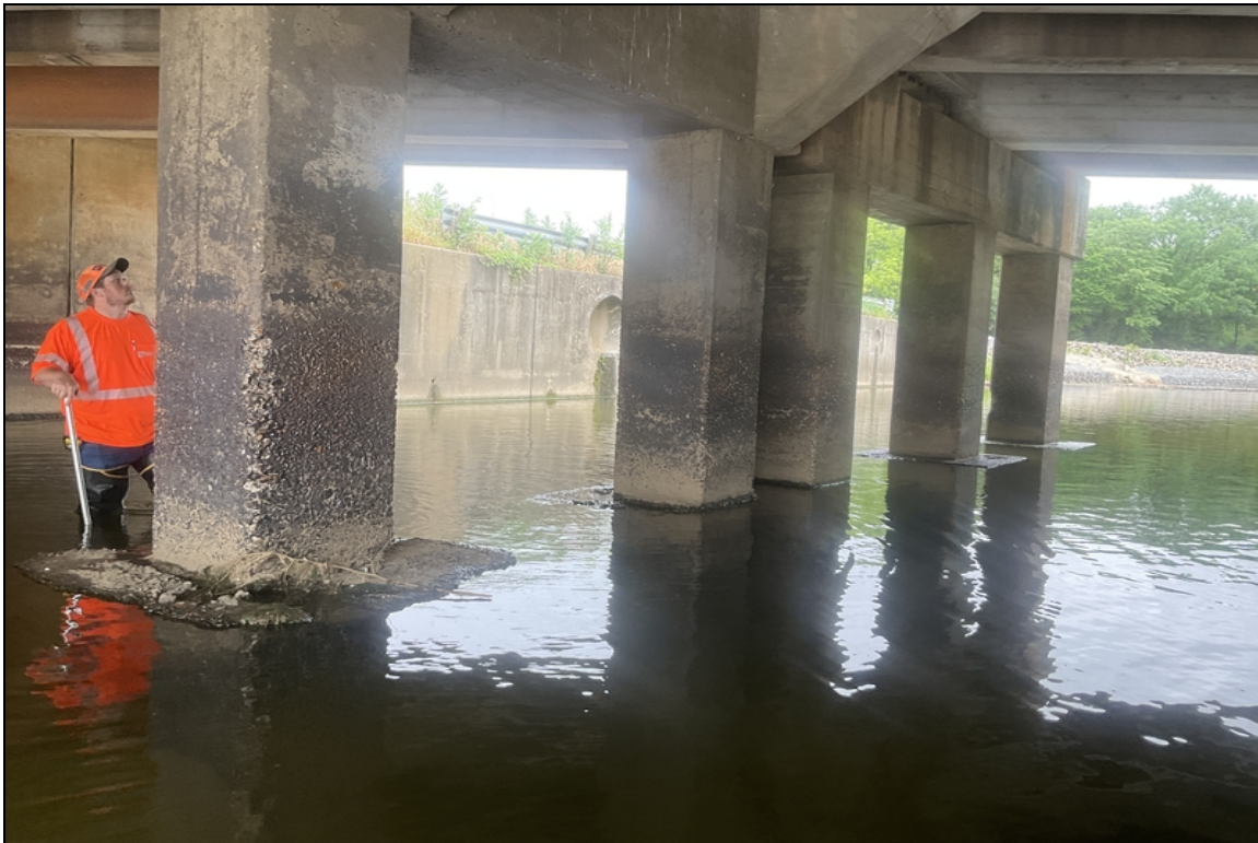
Substructure columns at Bent # 2. Typical.
