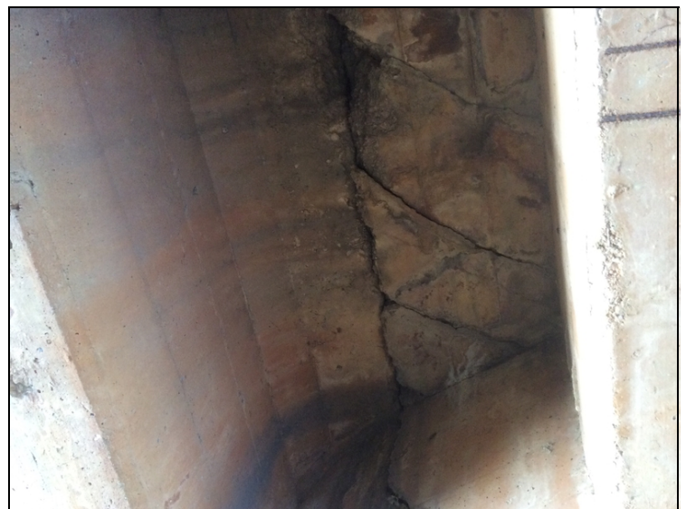
Span #1-Delaminated area in deck at construction joint over abutment #1.
