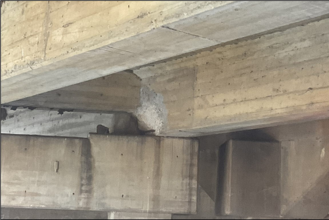
Span # 1 at Bent # 2 - Spall with exposed reinforcing steel in the end of Girder # 3.
