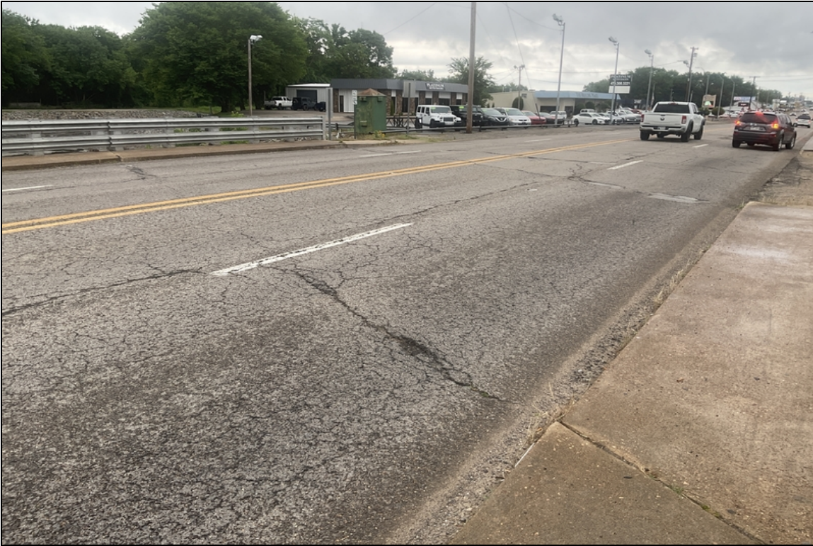
Asphalt breaking apart over the expansion joints with patched areas at the abutments.
