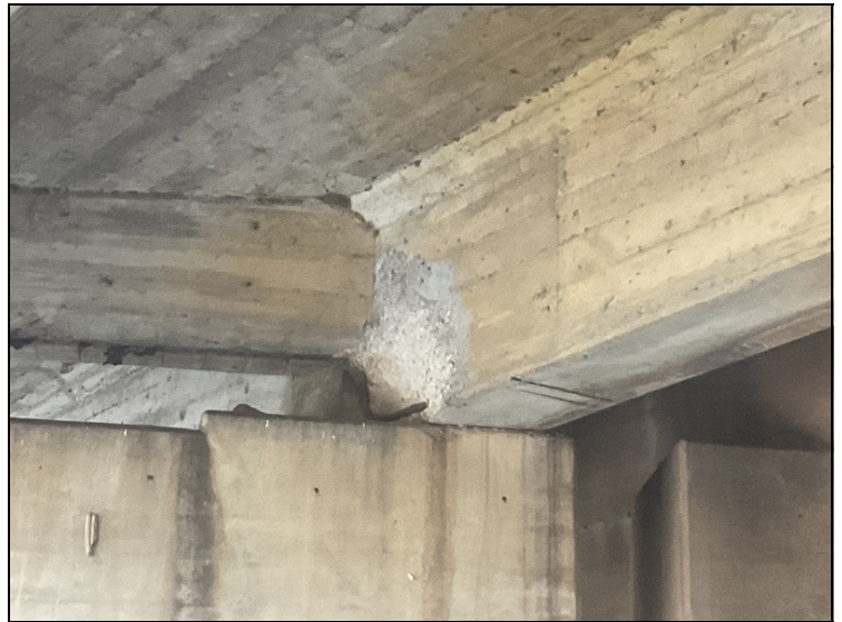
Span # 1, Girder # 3, at Bent # 2. Spall with exposed reinforcing steel.
