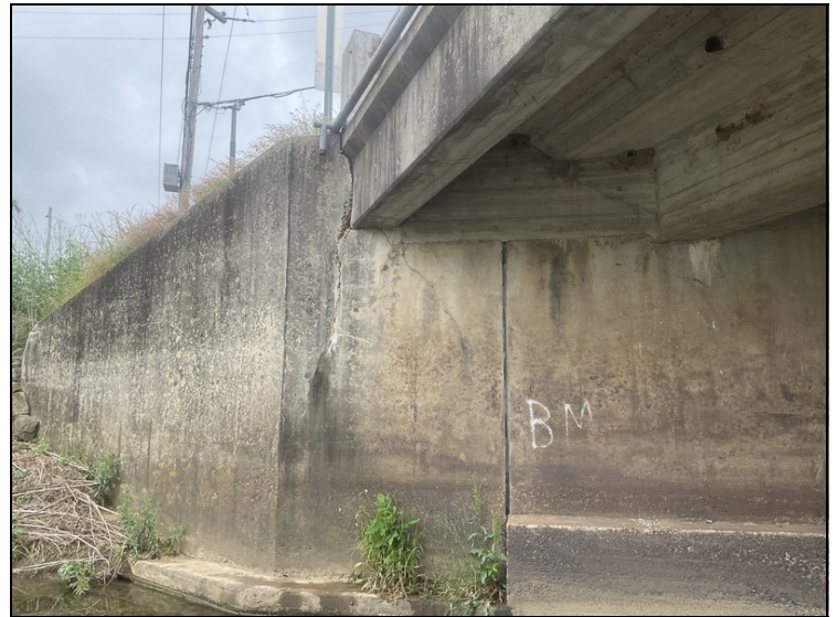
The Right side of abutment # 1 stem wall has diagonal cracking under girder # 9 with a 1/2 offset in the abutment stem (Appears to be delaminated).
