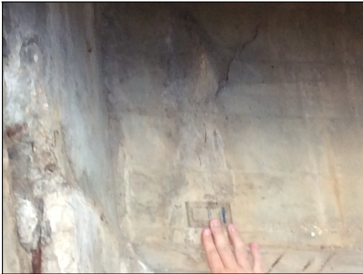
Shear Crack. Span 2, girder 7. Bent 3. Measures approximately 1/16" at this inspection
