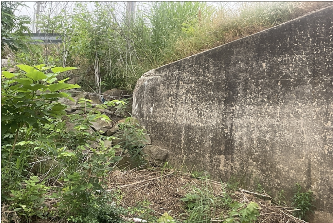
Bent # 1 Right end of the wing wall has concrete section loss and cracking with efflorescence.
