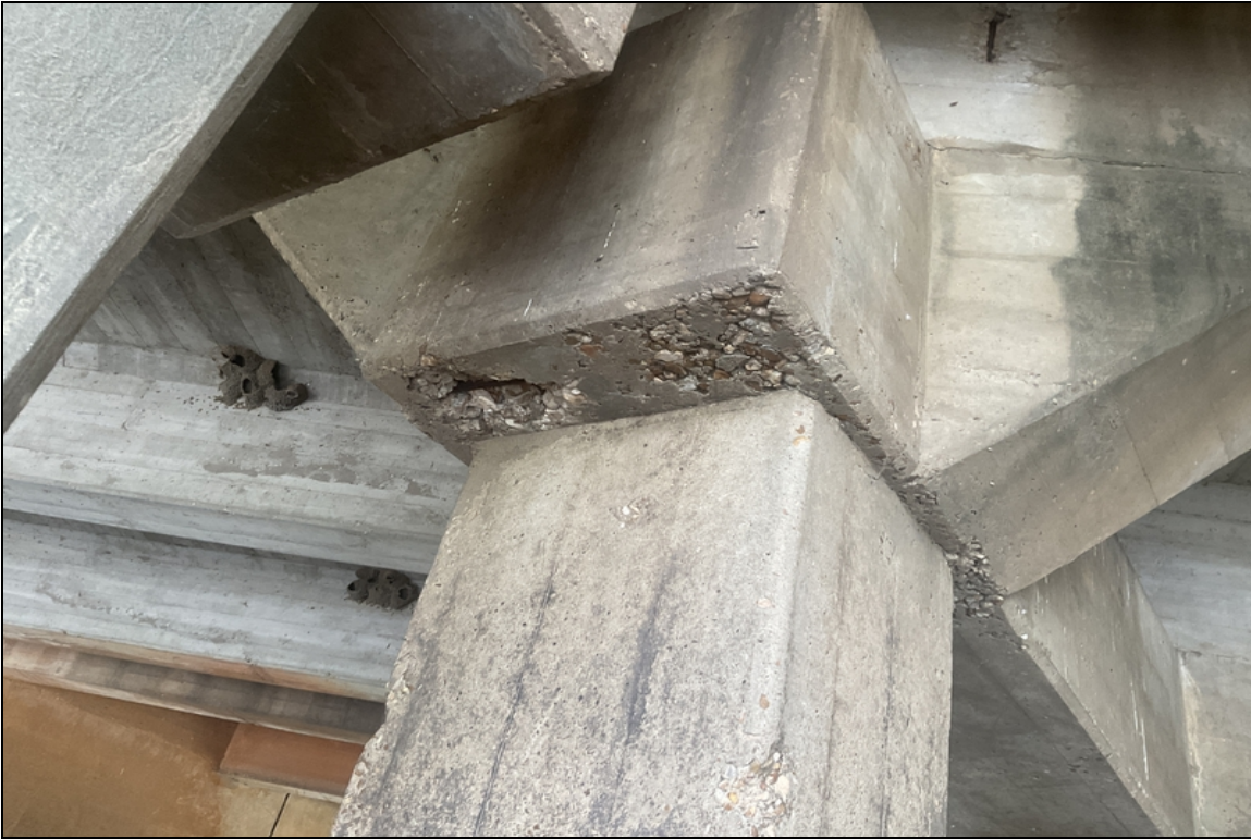
The undersurface of Bent # 2 cap has an 8" spall with exposed reinforcing steel adjacent to Column # 6.
