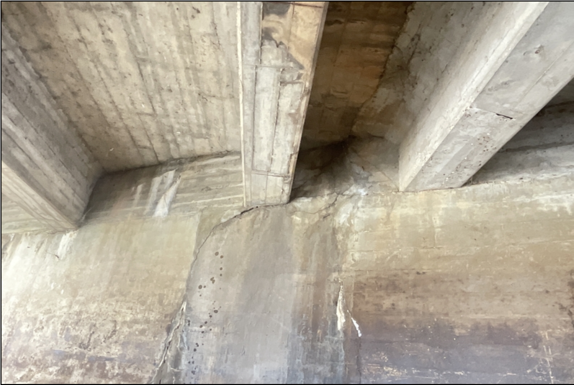
There is one 12" spall in the stem that has been patched between girders # 6 & 7 and adjacent to the Right side of Girder # 7.
