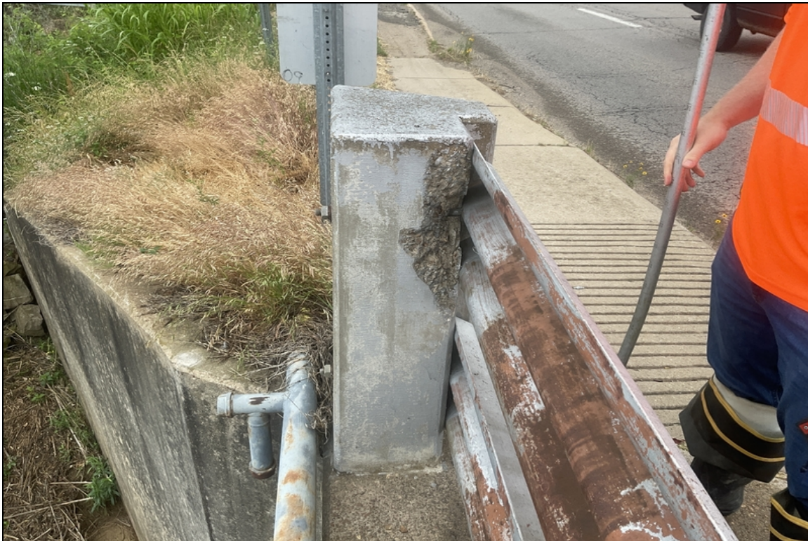
Spall with exposed reinforcing steel in the Southeast end post.
