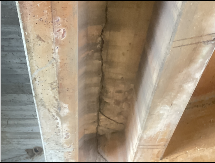
Delaminated area at the construction joint under Span # 1.
