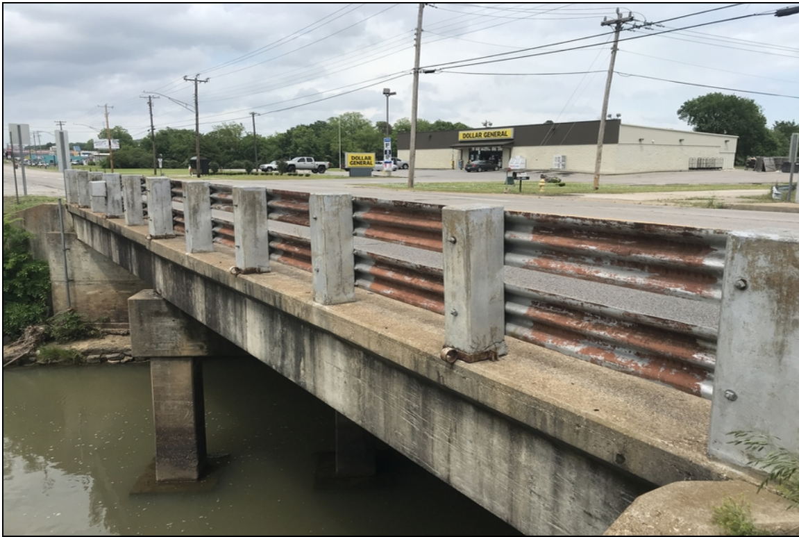
Typical backside of the metal bridge rail.
