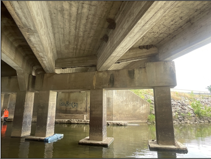
Bent # 2 cap has shallow spalling in the bearing areas of girders # 7, 8, & 9.
