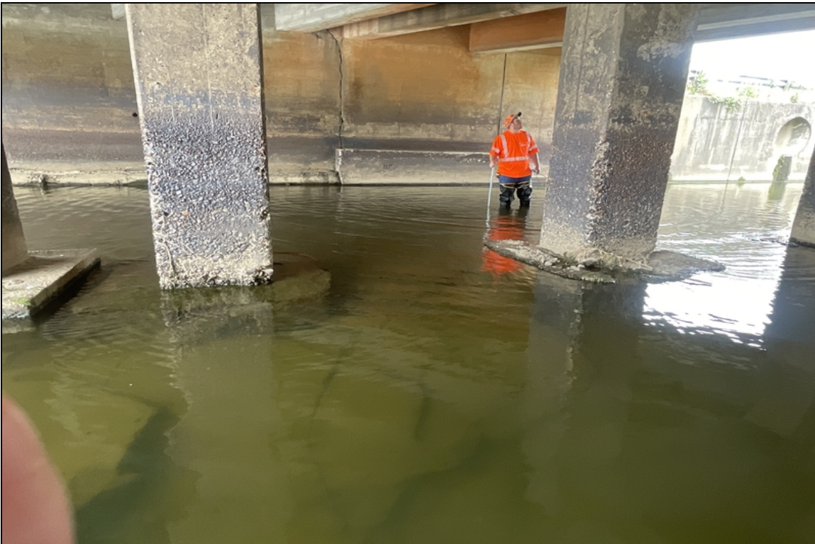
Concrete deterioration at the base of Columns # 5 & 6.
