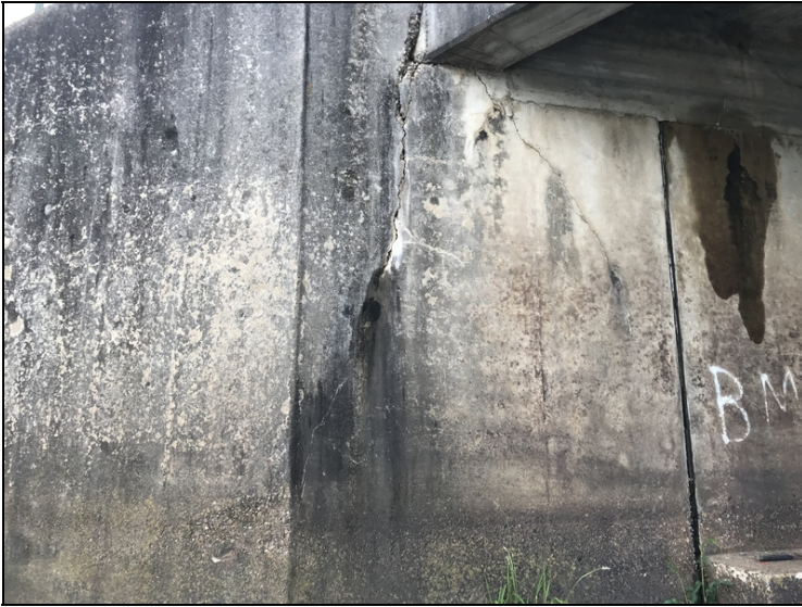
Bent # 1 Rt diagonal cracking under girder # 9 with a 1/2 offset in the abutment stem.
