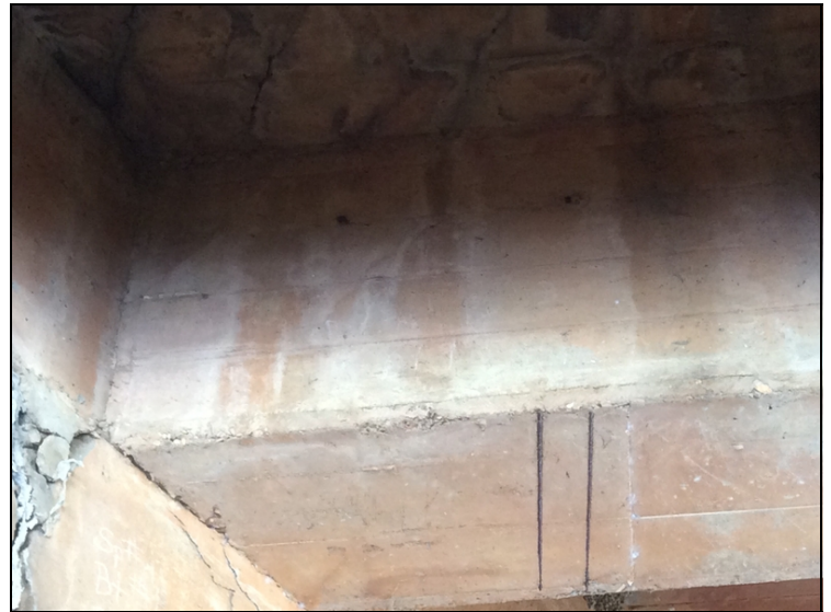
Hairline shear crack in Span 1. Girder 3. Bent 1.
