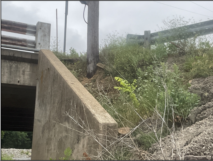
Embankment erosion behind the Northeast wing wall.
