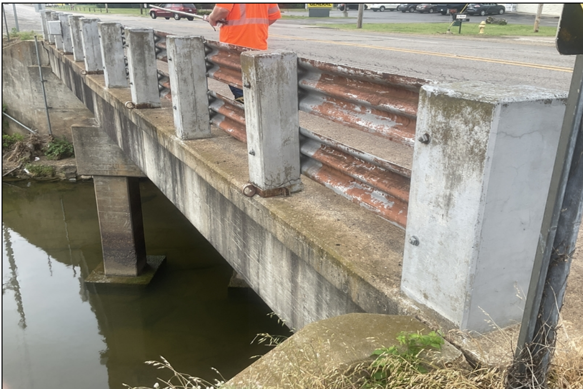
Span # 1 Left side. Fractured concrete bridge railing post.
