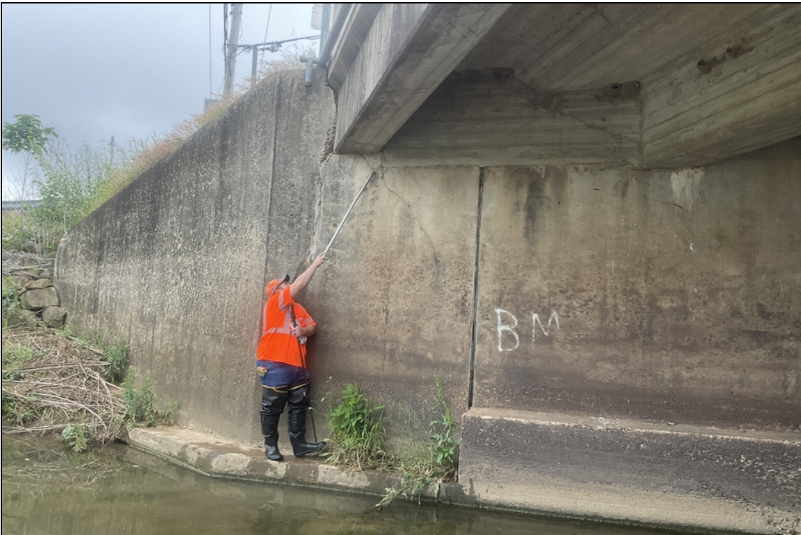
Bent # 1 Right has diagonal cracking under Girder # 9 with a 1/2" offset in the abutment stem (appears to be delaminated).
