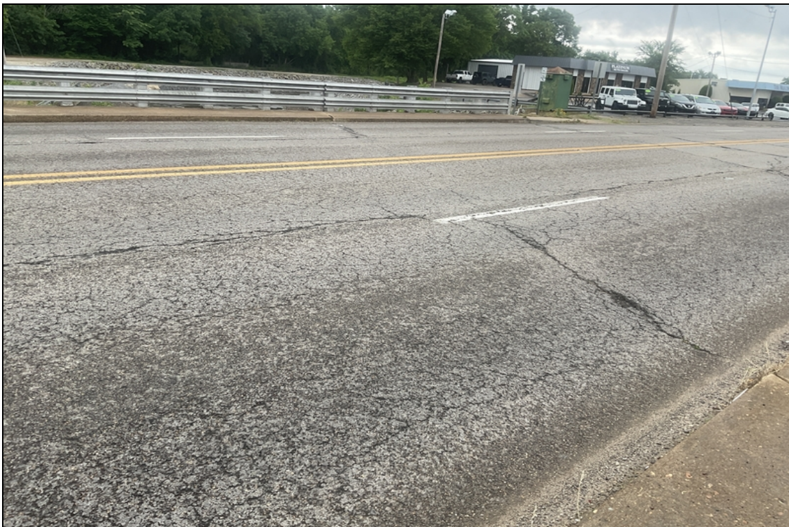
Asphalt breaking apart over the expansion joints.
