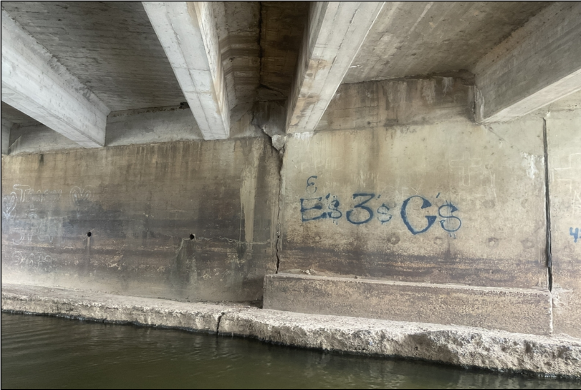
There is a 3' spall with exposed reinforcing steel in the vertical construction joint between Girders # 6 & 7.
