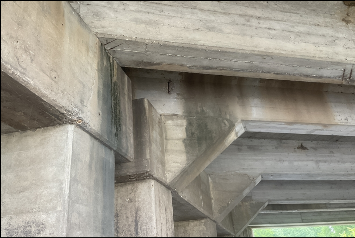
Span # 2 Girder # 6 has a 8" vertical spall with exposed reinforcing steel adjacent to Bent # 2.
