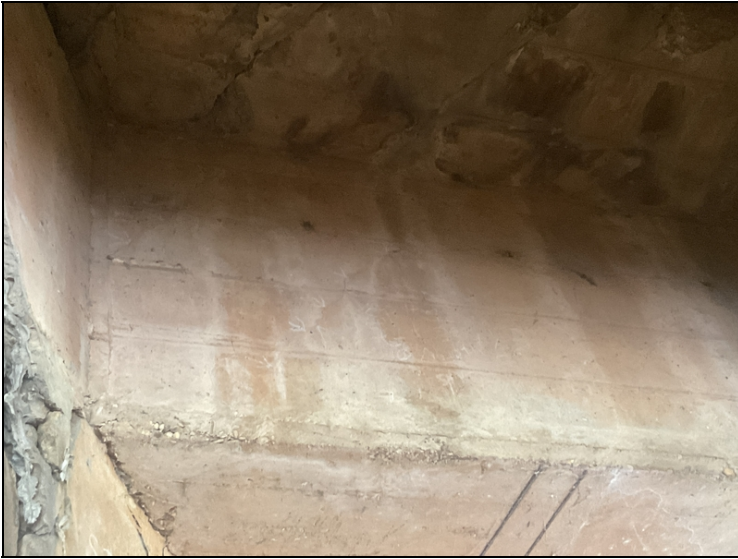
Span # 1, Bent # 1, Girder # 3, hairline shear crack.
