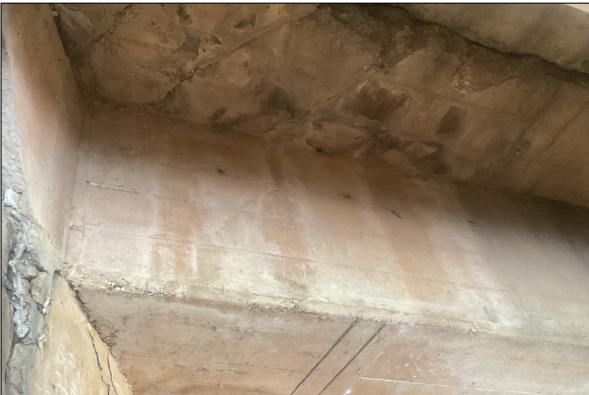
There is one hairline shear crack in Girder # 3, Span # 1, adjacent to Abutment # 1.
