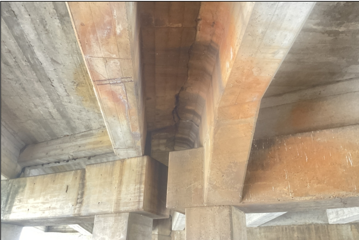
Spalling in the deck soffit over Bent # 2, Bay # 3.
