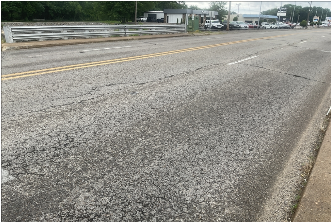
Decks Typical. Asphalt wearing surface has map cracking.
