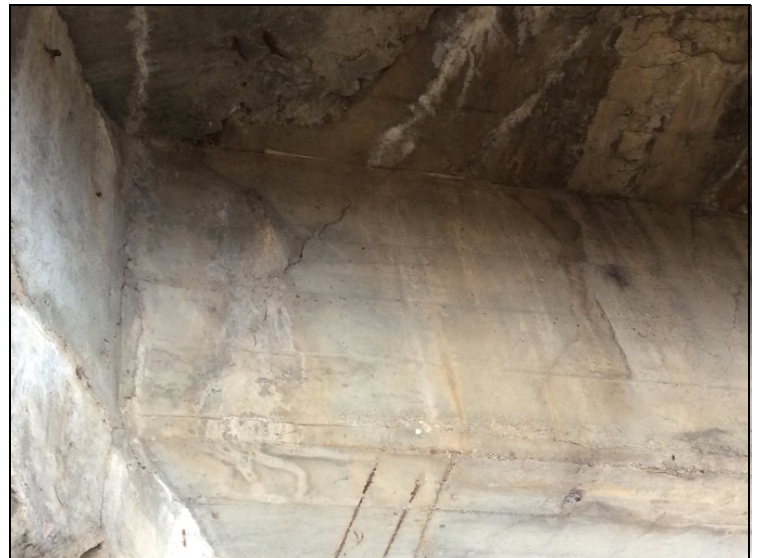
Open shear crack. Girder 7. Bent 3.
