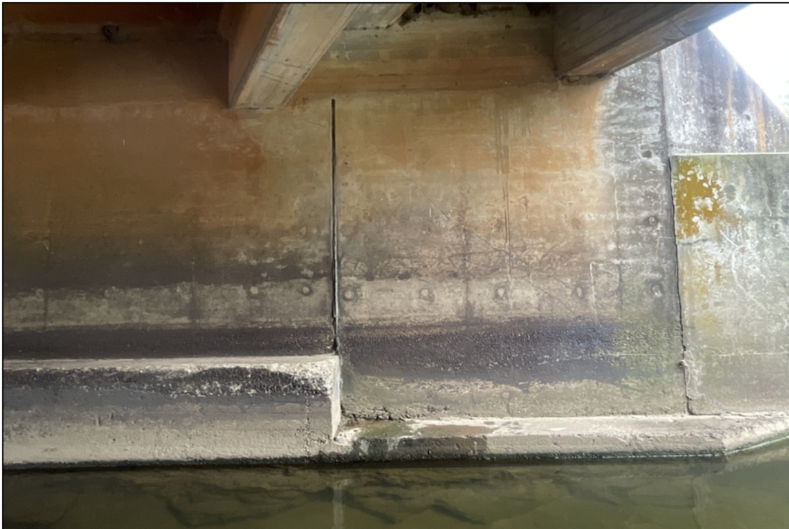
Bent # 1 Left has a 9' long X approximately 1/16" wide diagonal crack under Girder # 2, Bay # 1.
