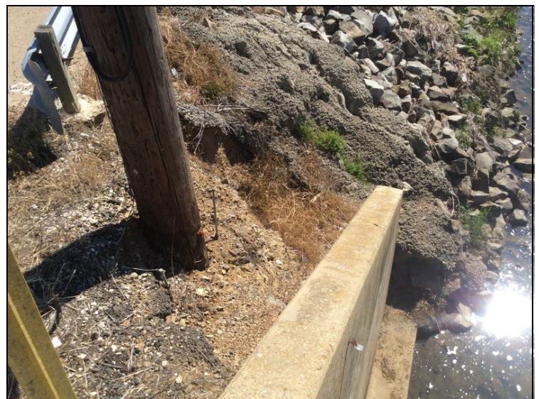
Minor erosion behind Northeast wing wall.
