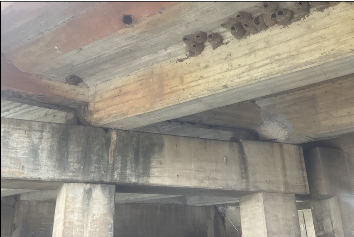
Span # 1, Girders # 2 & 3 at Bent # 2 - Spalls with exposed reinforcing steel.
