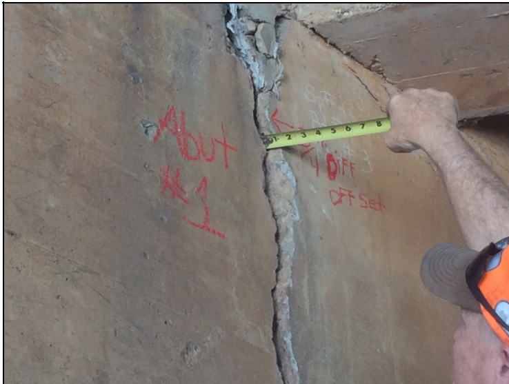
End Bent 1-Differential offset in stem wall.
