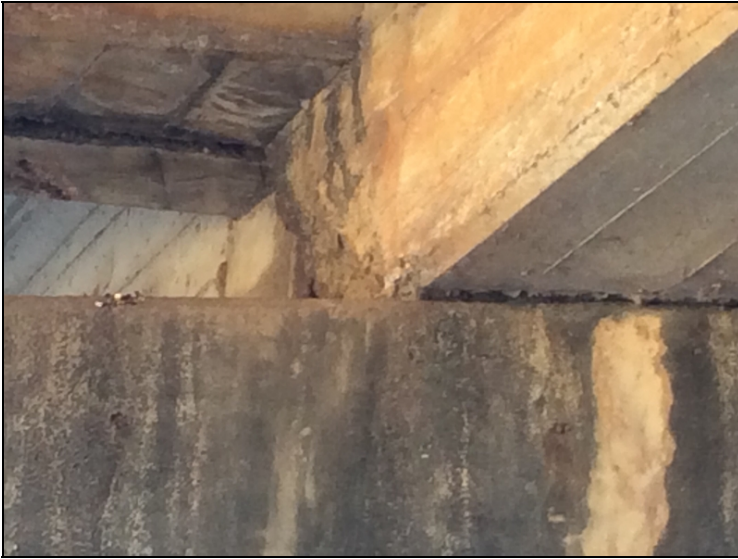
Span 1, girder 2 over Bent 2-Spalling.
