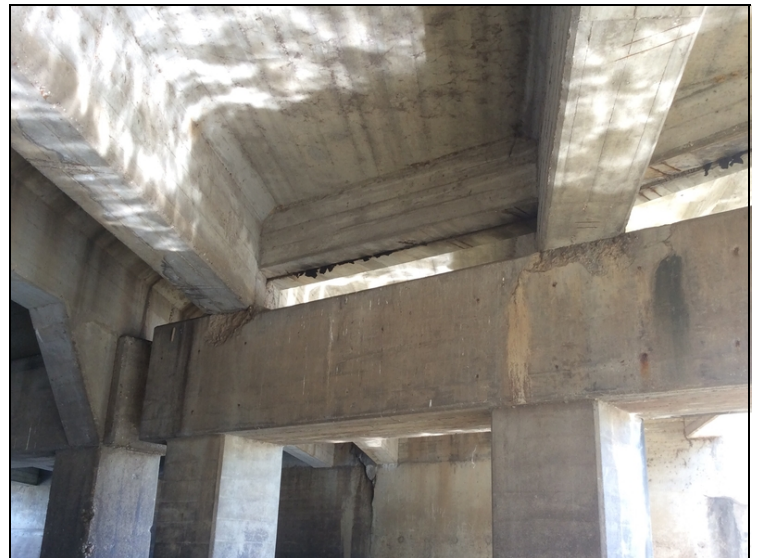
Bent #2 cap-Spalling in bearing area of girders #7 and #8.
