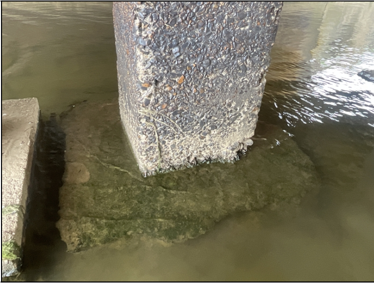
Concrete deterioration at the base of Bent # 2, Column # 6.
